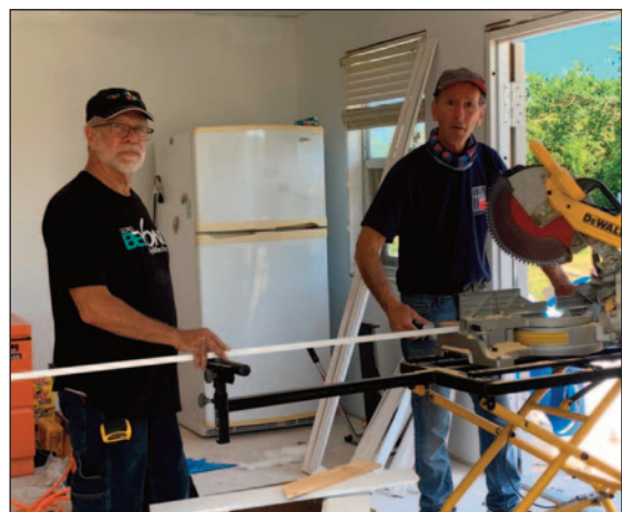
Door and window installation
