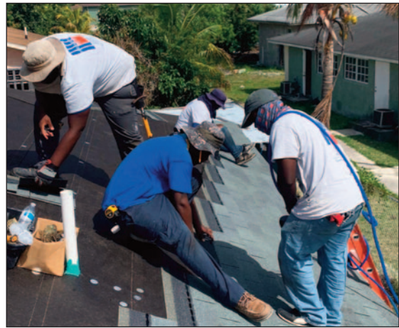
Hurricane Dorian Pre-Apprentice Class 2 roofing
