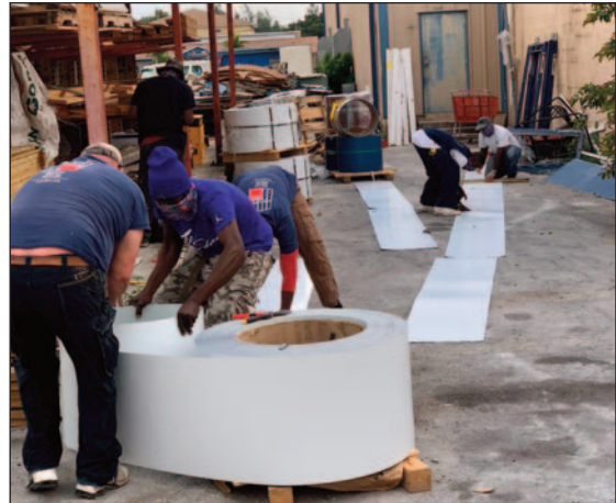
Hurricane Dorian Pre-Apprentice Class 2 picking up roofing material
